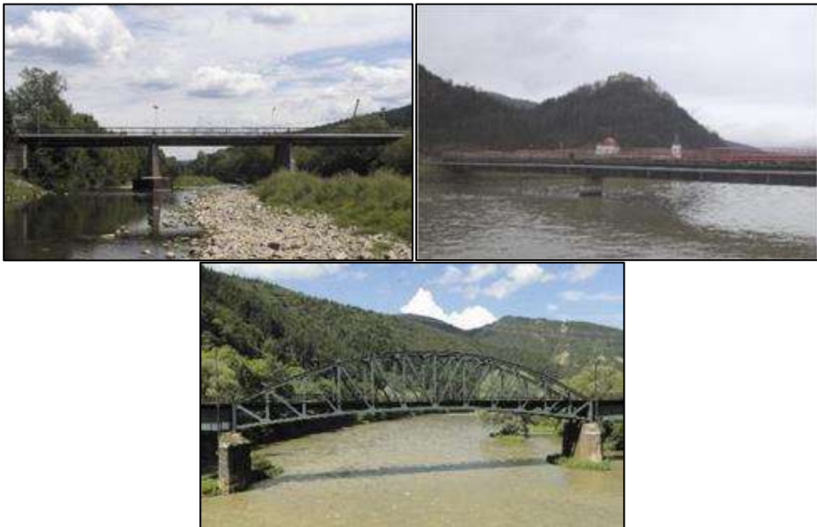
Fig. 4: a) the road bridge A across a river; b) the bridge B on a local service road across a river canal; c) the railway bridge C across a river.
